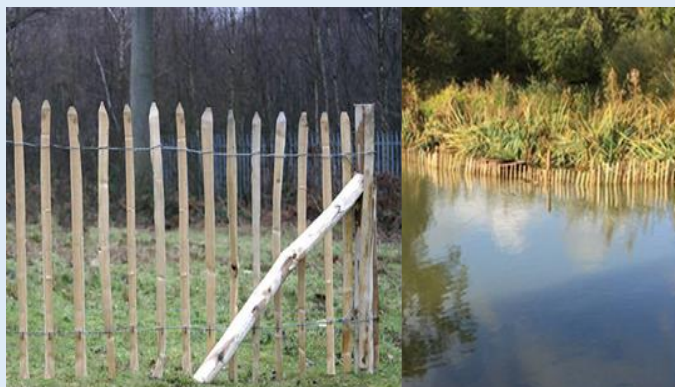
Submerged chestnut piling has now turned this reed fringe from a dinner table into a sanctuary area.
